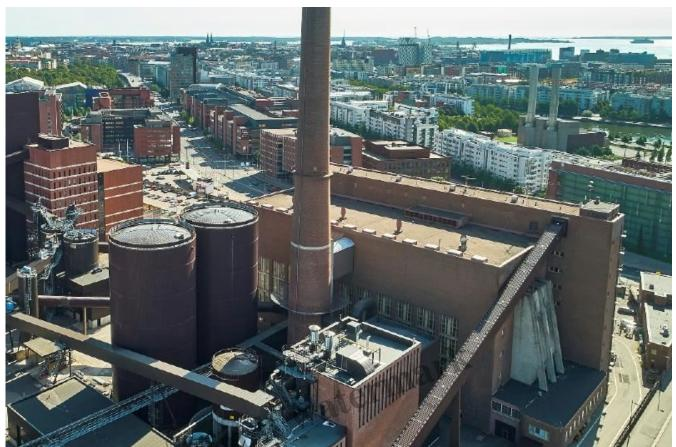
Valmet is to convert Helen Ltd's coal-fired district heat boiler to bubbling fluidized bed (BFB) combustion at the Salmisaari power plant in Helsinki, Finland.
